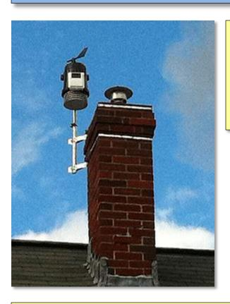
**LEFT:** Station notes indicated that this is an inactive chimney, but the temperature and humidity sensor is still too close to the black tar shingle roof. The brick also is likely to radiate heat.
