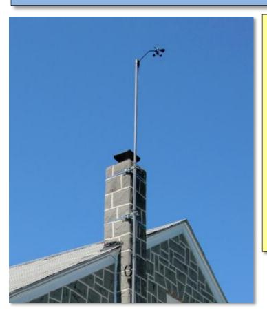
**LEFT:** Chimneys can provide a nice, solid structure for mounting an extension pole. Chimney mounts designed for antennas can be purchased in most home improvement and electronics stores.
