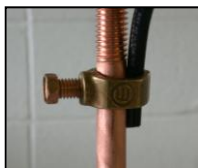
Figure 19: The #4 cable connected to the ground rod.
